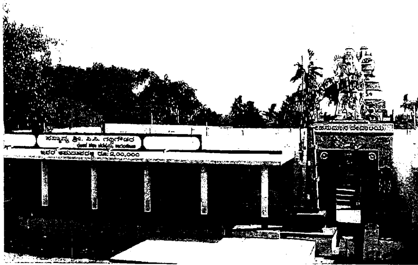
Figure 7.1 Community Hall Constructed with MPLADS Funding, Bagalkot District, Karnataka State, 2008–09. Source: GOI (2010: 90).
